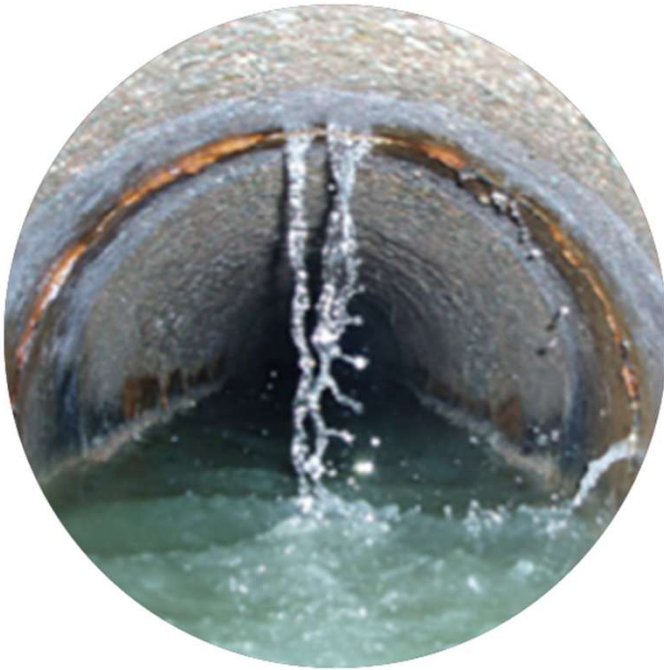
Example of Infiltration into a Sanitary Sewer
