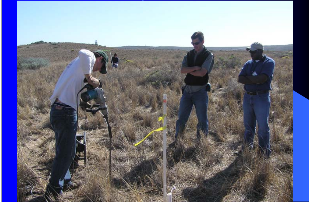
Hammering a hand-probe in the ground with a rotohammer.
